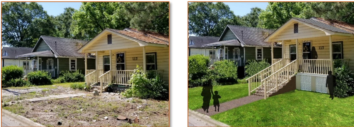
Figure 18: Rendering of home before (left) and after (right) being elevated.
