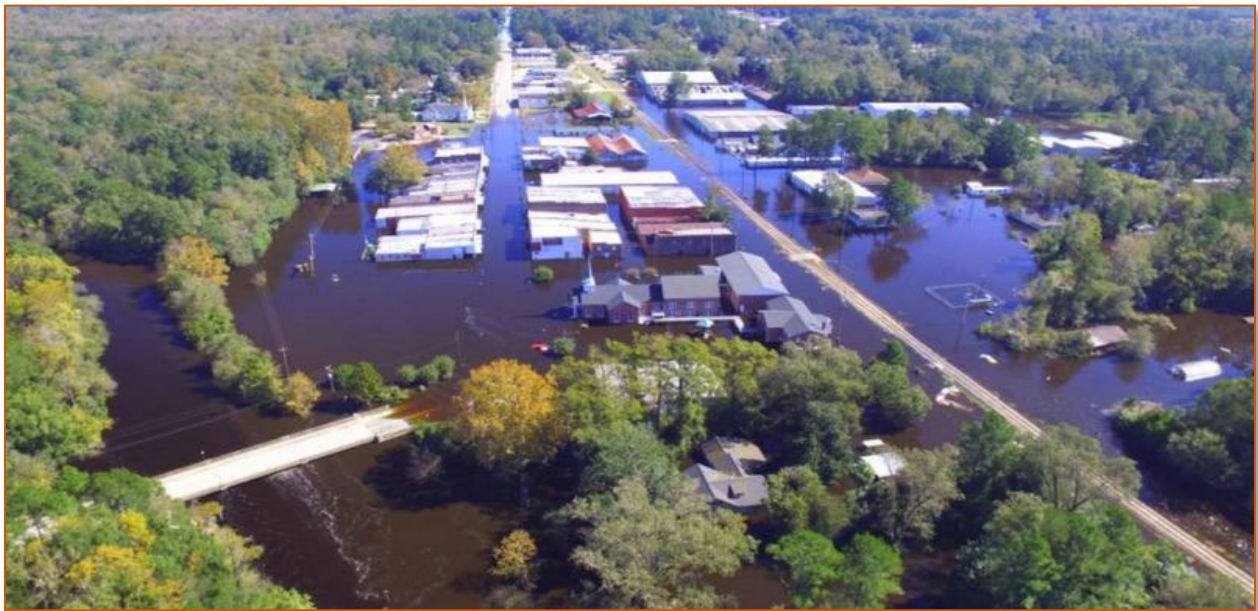
Figure 22: Downtown Fair Bluff flooding following Hurricane Matthew.
