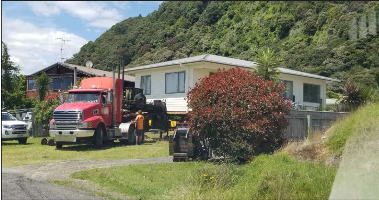
Figure 6.2 House in Matatā being prepared for relocation (Photo: G Smith).
